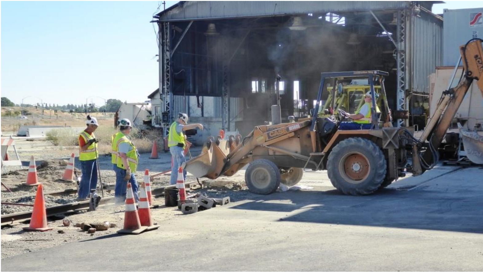
Harry on the back-hoe brings in more rock to fill-in along the field-side of the rail
