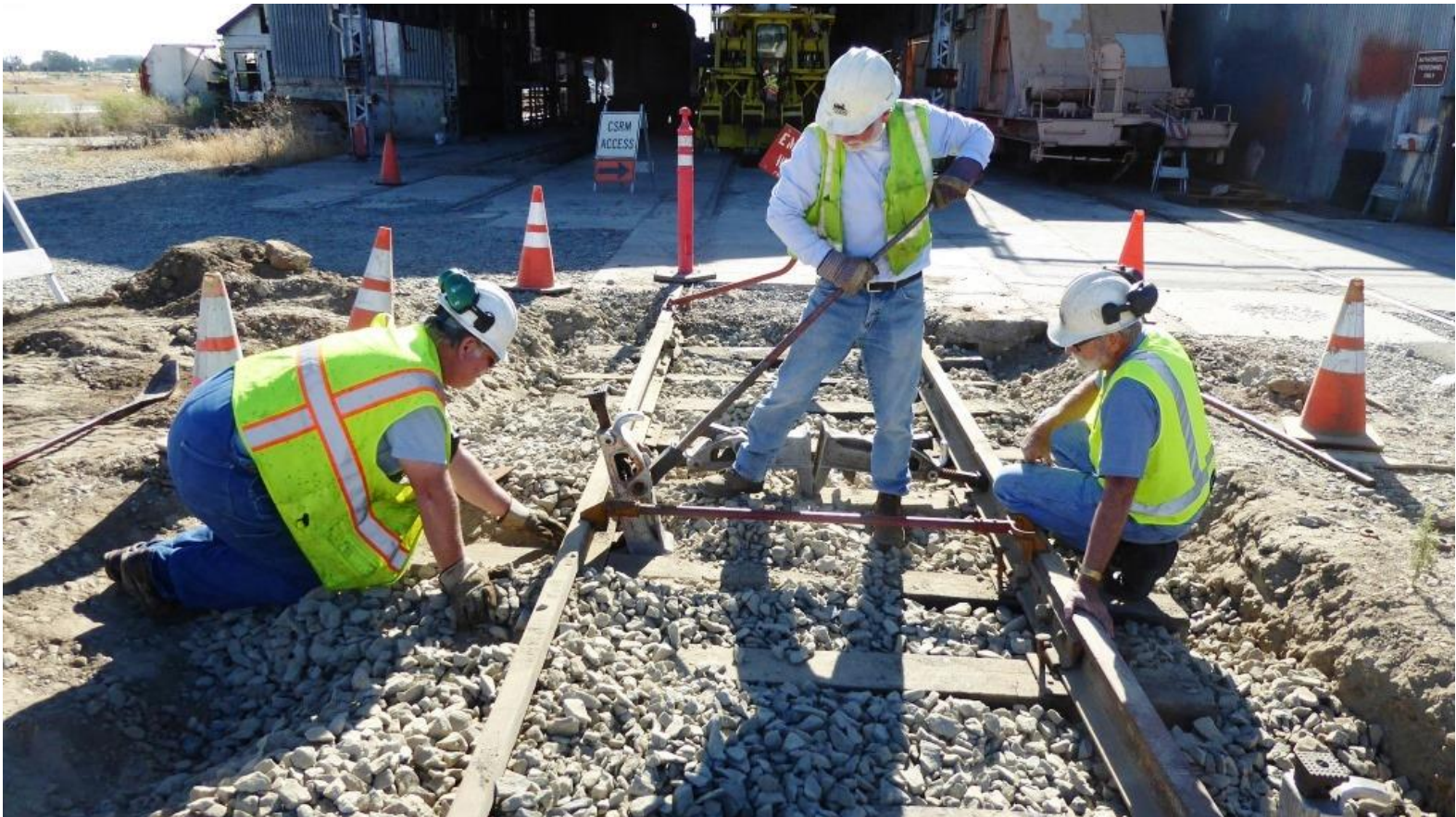
Mike M. cranks on a track-jack to lift the rail slightly so that a tie-plate can be placed
