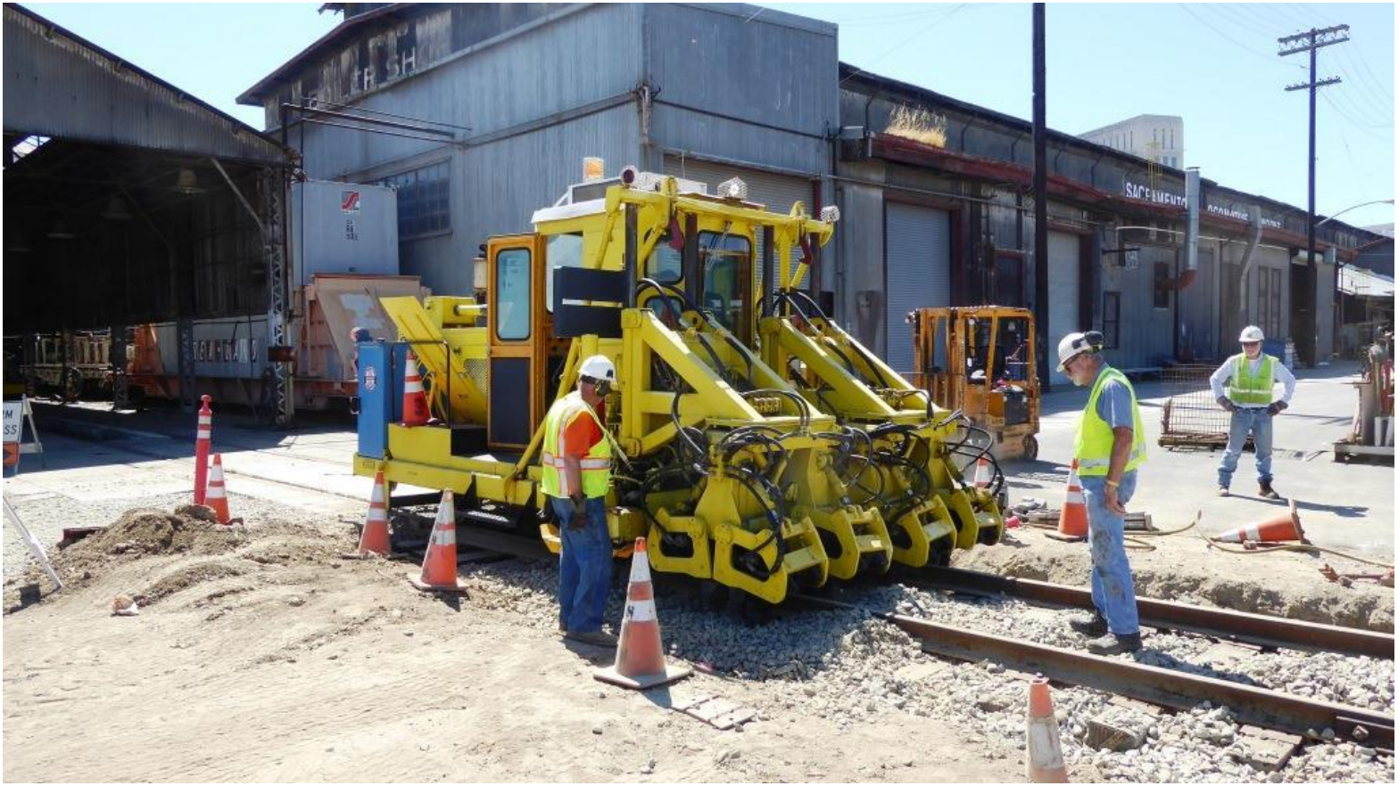
The work-heads descend deep into the ground around the tie to squeeze rock under it
