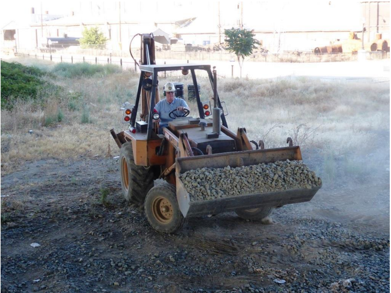
Chris gets a bucket-load of ballast rock for the Firing Line extension track
