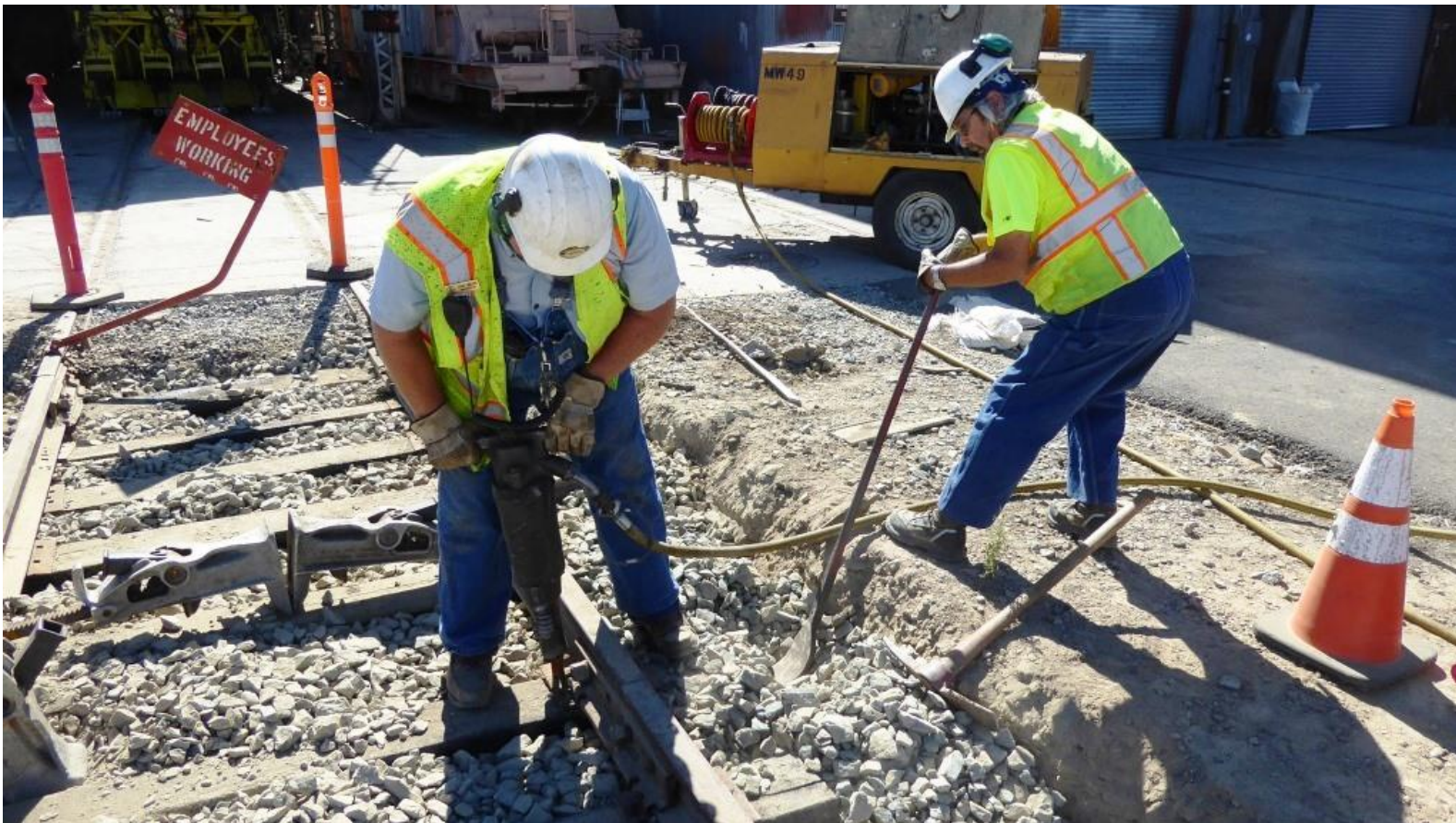
While Ed nips-up the tie, Chris drives a spike with the 90-lb. pneumatic spike-driver
