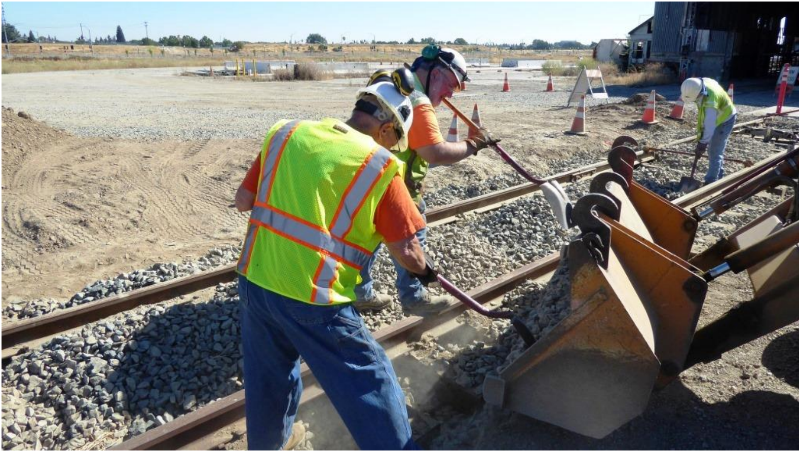
Clem and Frank pull rock out of the back-hoe's bucket to fill-in around the ties
