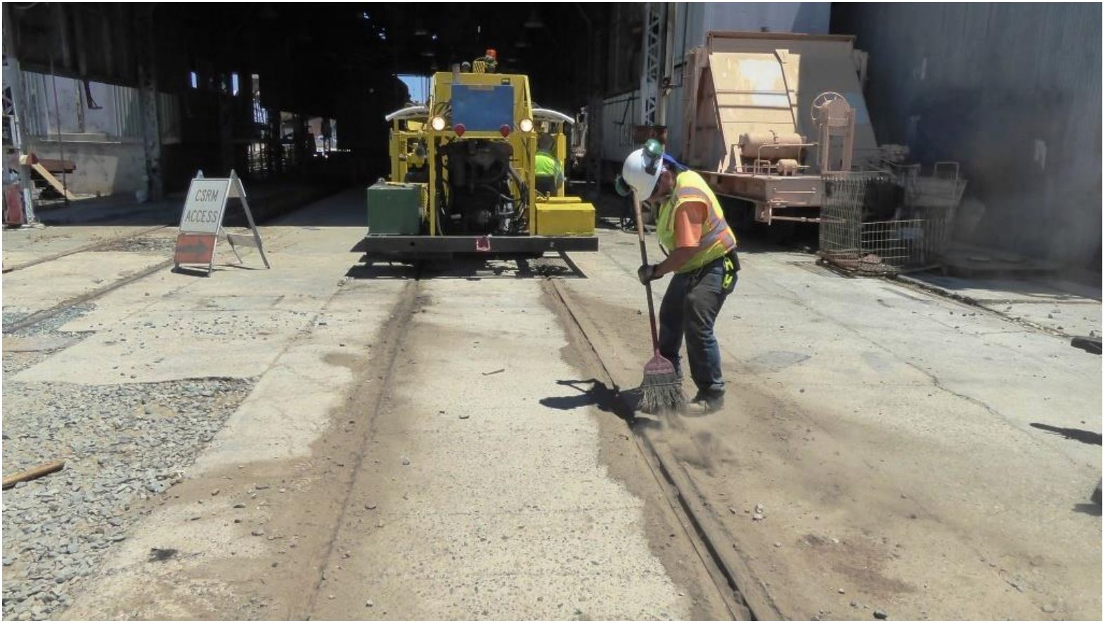
Joe clears the flange-ways of the old Firing Line track to remove any impediments that might impede the spiker's progress
