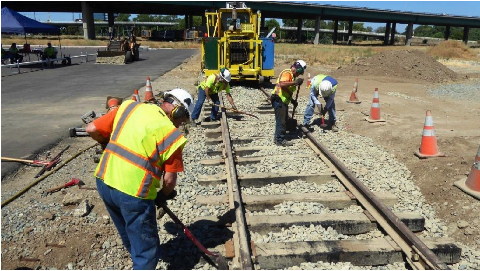
After the initial tamping, Clem, Ed, Joe, and Mike M. work behind the tamper to add more rock for the next round
