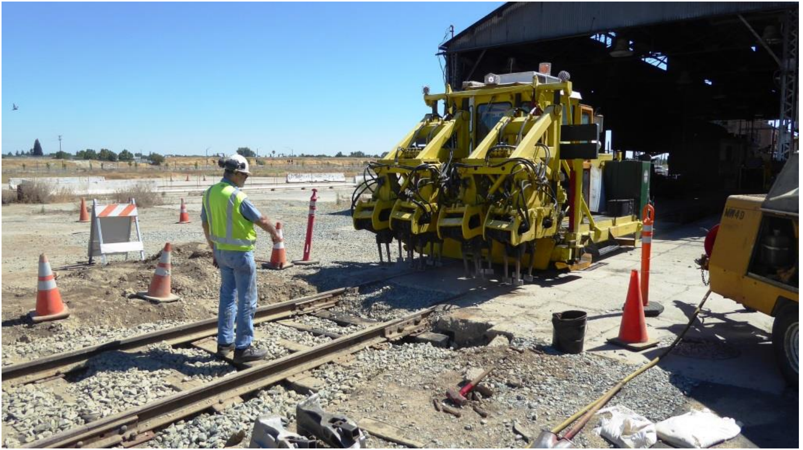
Time to tamp! Chris brings in the tamper as Alan provide direction from the ground
