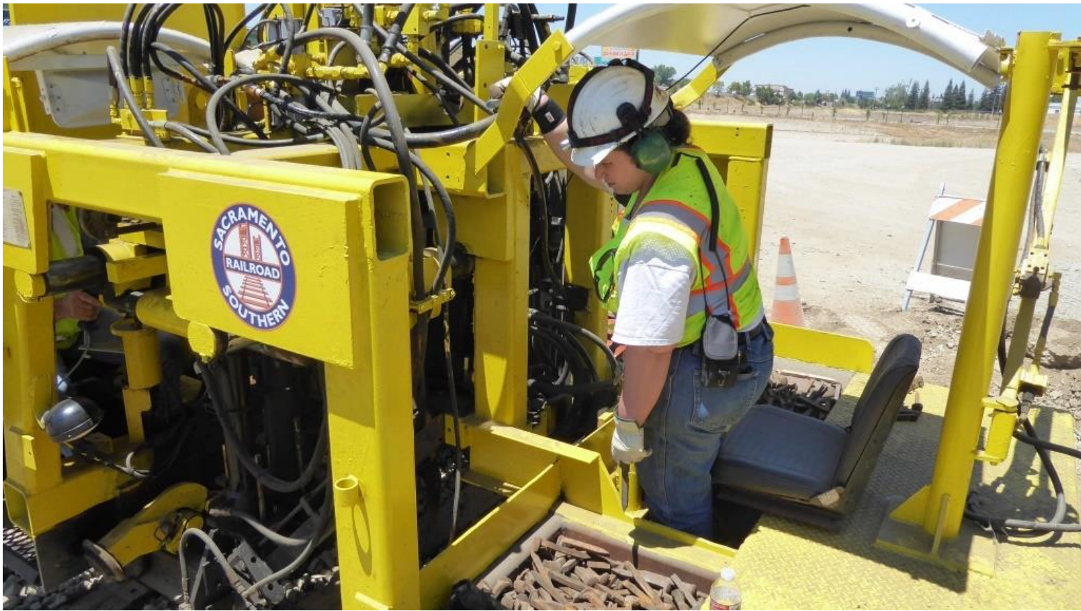
Heather operating the system that feeds the spikes to the spiking rams
