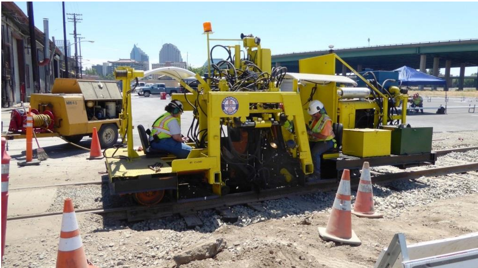
Heather, Joe and Alan soon get the routine down and get the rest of the ties spiked with the spiker
