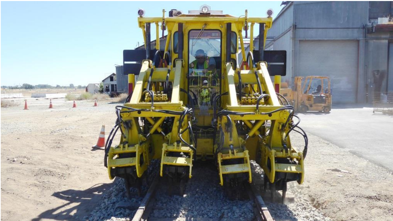
Chris at the controls of the tamper
