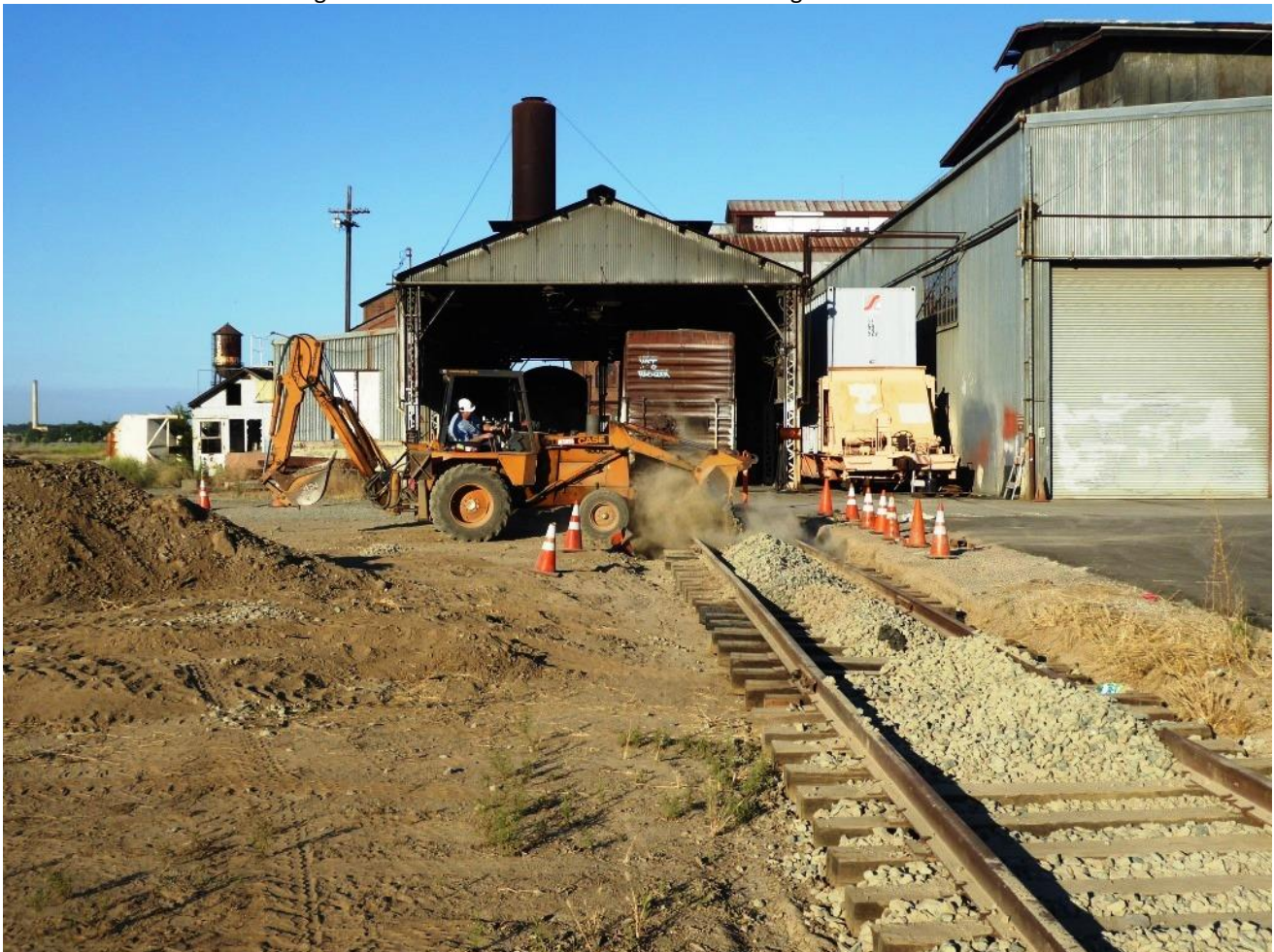
Chris moved 15 loads of rock to the extension track on Thursday evening
