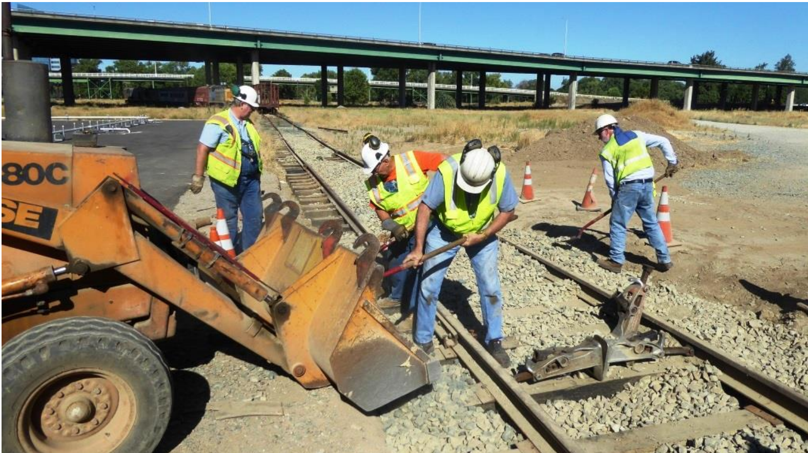
Alan and Clem engage in some precision ballasting
