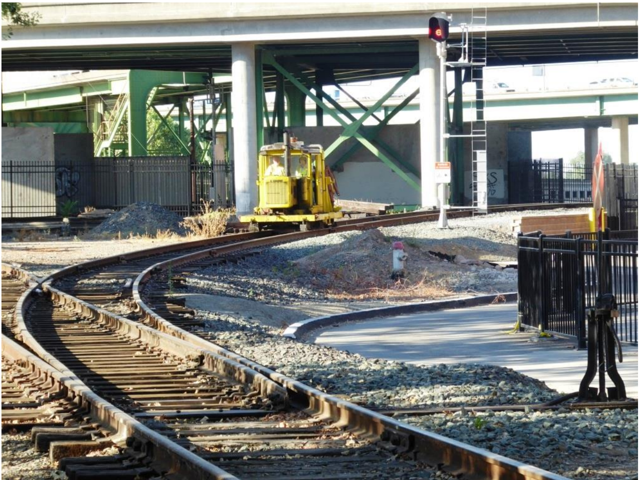
Engineer Weston and Conductor Frank bring the Kalamazoo over from the Shop
