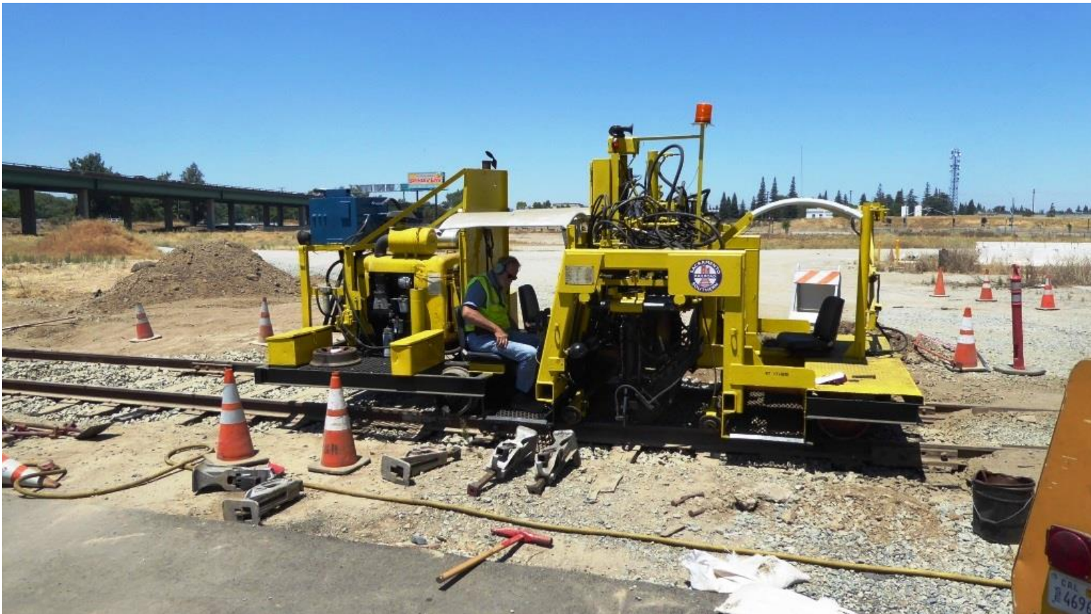
Alan at the controls of the spiker
