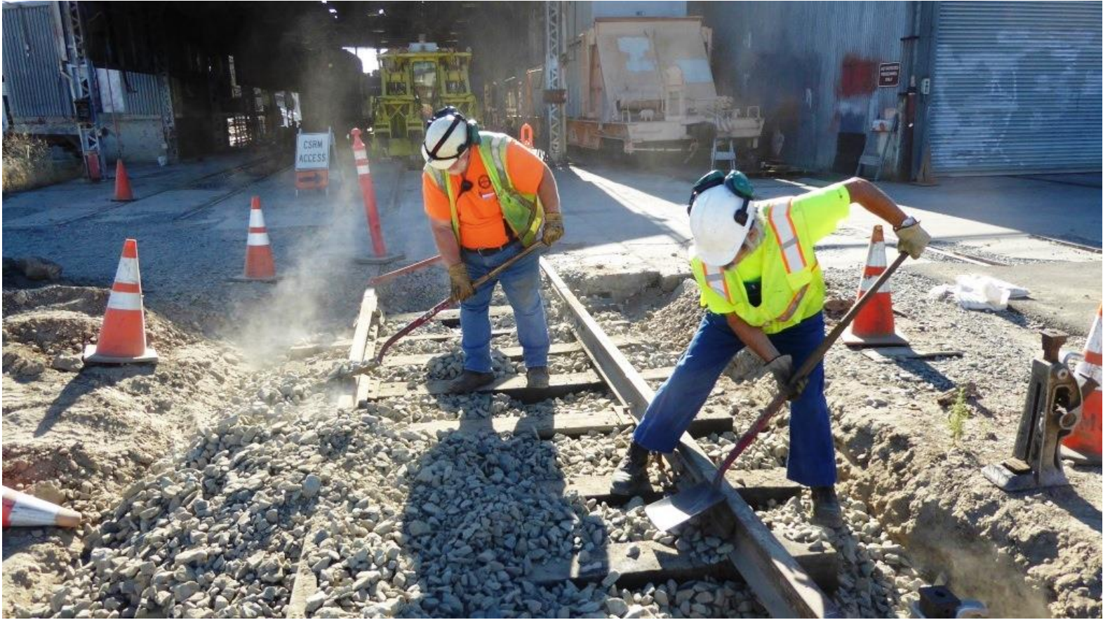
Frank and Ed moving ballast-rock about to fill-in holes and spread it evenly
