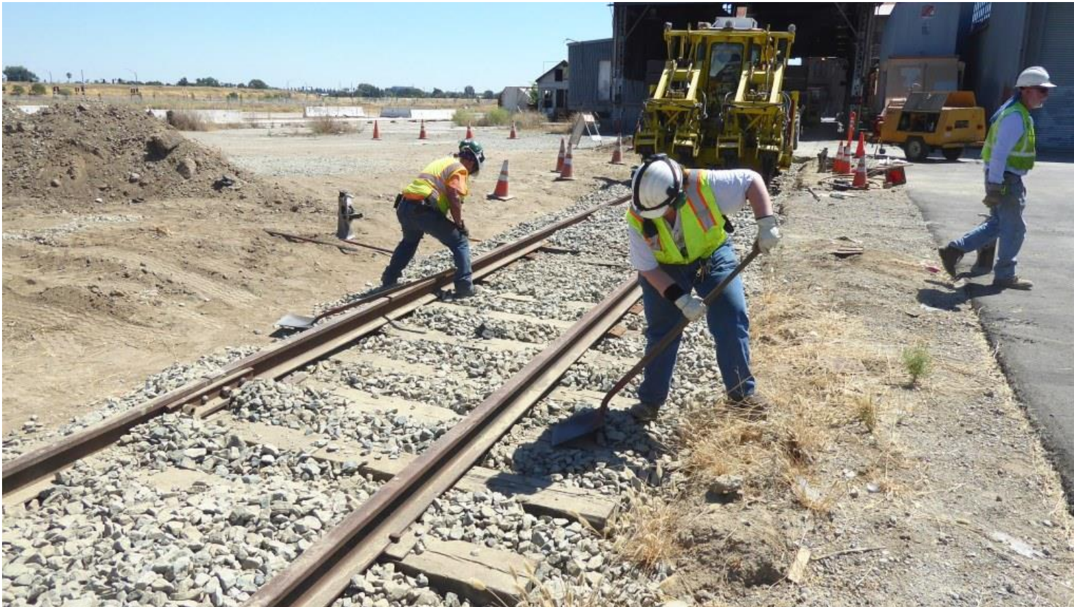
Heather and Joe work ahead of the tamper to make sure there's plenty of rock to be squeezed under the tie
